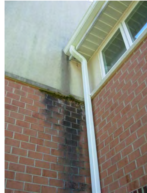
2. Gutter leaking causing organic material growth
