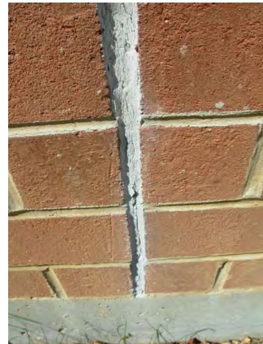
4. Drying and cracking of vertical control joints
