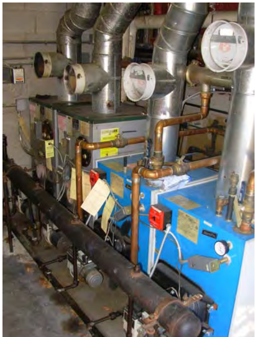
7. Heating and DHW generation boilers
