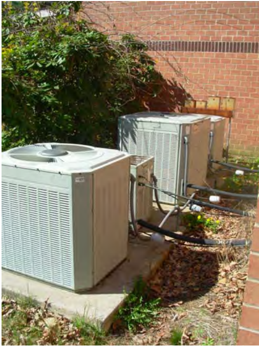
9. HVAC split system exterior condensers
