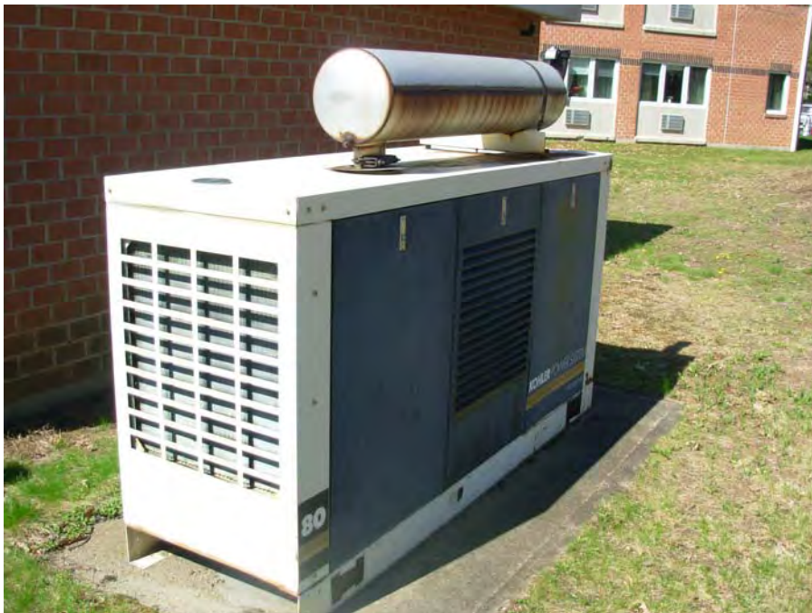
11. Emergency generator, due to be overhauled
