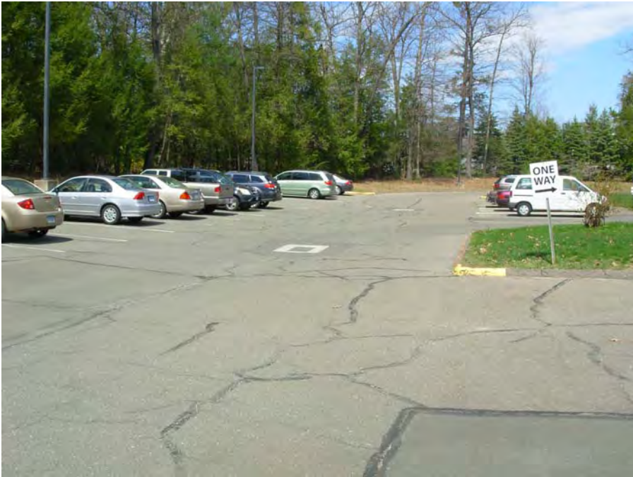
1. Sporadic cracking of asphalt paving
